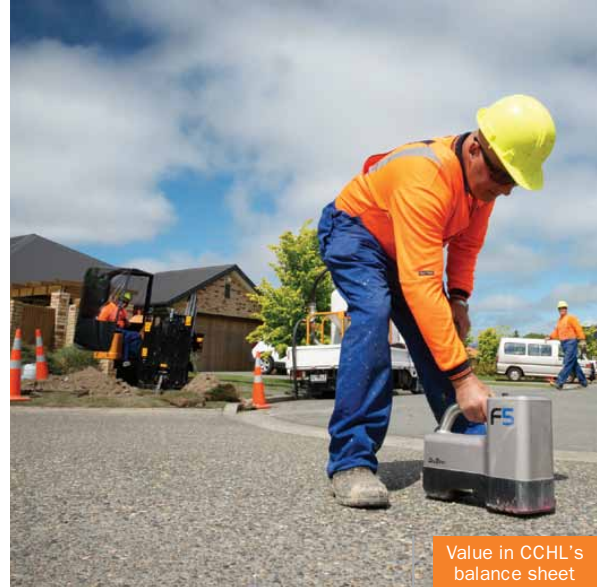
ESL contractors deploying fibre broadband in a Christchurch suburb.
