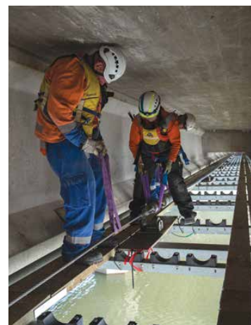
A Connetics team laying cables under the Bridge Street road bridge.
