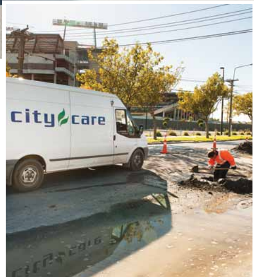
Above: City Care crew works on jetting a sewer line and then sucking the silt from the sewer as it is drawn back to the manhole.
