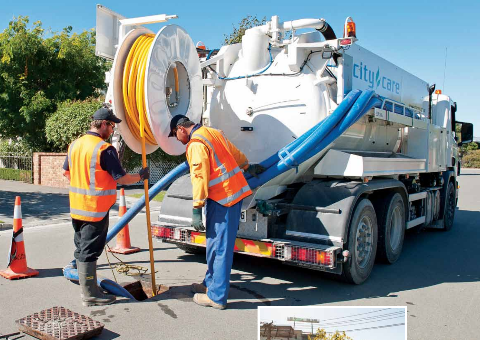
Above: City Care crew works on jetting a sewer line and then sucking the silt from the sewer as it is drawn back to the manhole.
