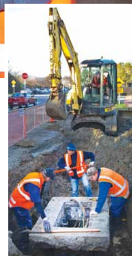
Above: Enable contractors splicing fibre cables to connect Lyttelton to Christchurch.
